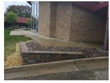
If you haven't noticed, a new retaining wall was constructed just to the north of the parking lot entrance. This new wall was installed to prevent further erosion under the sidewalk and to provide for a safer walkway area. During the week the entrance to the church is through the courtyard and the doors near the office.
